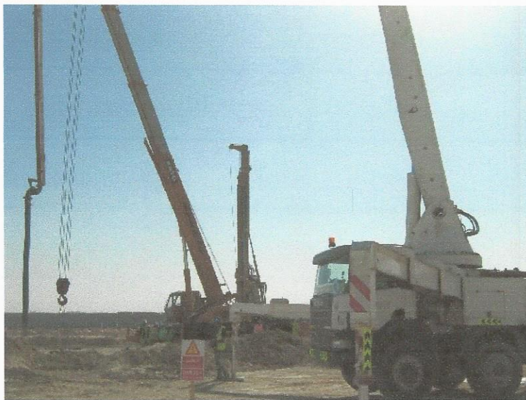
1200 MM. DIAMETER BOREHOLE FOR GEOTHERMAL PLATFORM & INSTALLATION OF 18 METERS OF 1016 PERMANENT CASING
